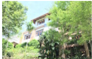
Shambala Estate Renovation, Samui
